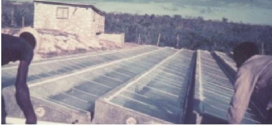
Solar still serving a village in Haiti. This still has an area of about 300 m 2 (3,000 ft 2 ). It was put in operation in about 1967 and was reported as operational in 1998. Photo — Brace Research Institute
