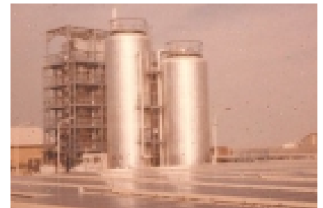
This MED unit in the United Arab Emirates has operated since 1985. The evacuated tube solar collectors in the foreground provide heated water input for the unit. Its design output is 80-m 3 /d (0.02 mgd).
