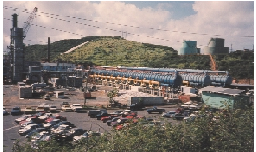
Three low-temperature MED plants on St. Thomas (VI). Each plant has a capacity of about 5,000 m 3 /d (1.2 mgd). Photo — OK Buros
